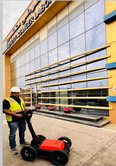
AHSL UAE now forays UNDERGROUND to assess Utilities with their brand New GPR (Ground Penetrating Radar)
