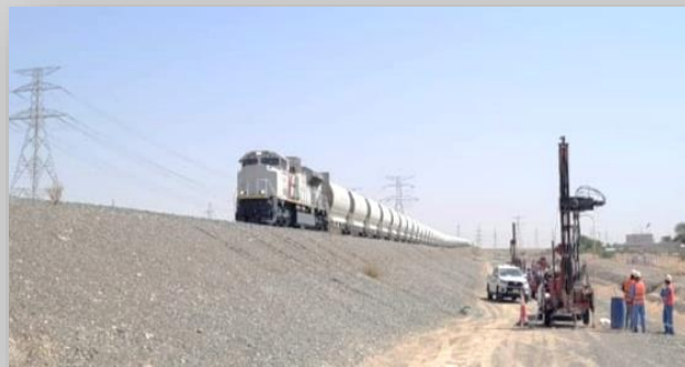
GT works ongoing in the vicinity of Etihad Rail, AUH
